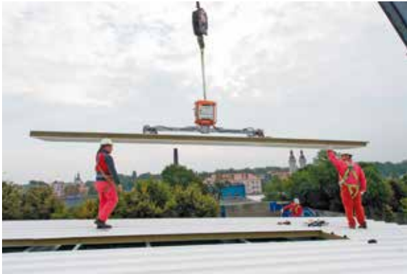
Pic. 8 and 9. Assembly of roof panels.
